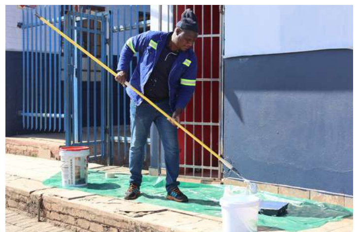
Armscor employees repainting classrooms at Meetsing Primary School.
