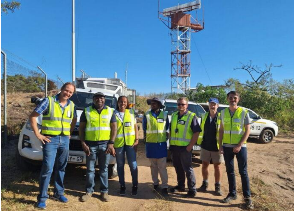
ATNS and the CSIR are installing passive radar technology at KMIA.
